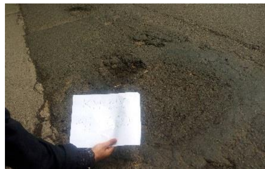
Patching and Utility Cut Patching
